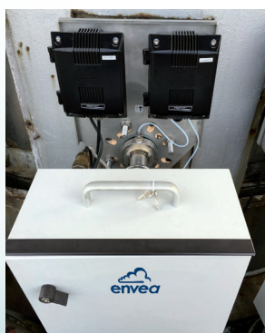
Combined version : Gas sample & FTP measurement on a same flange
