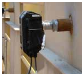
ElectroDynamic™ sensor installation in multicompartment baghouse
