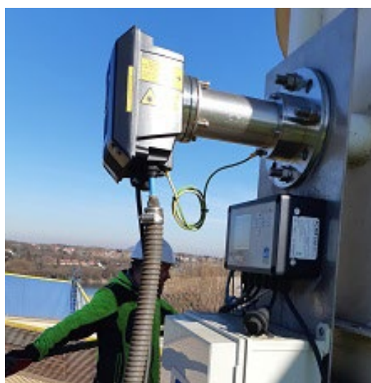
ProScatter TM Particulate CEMS Installation
