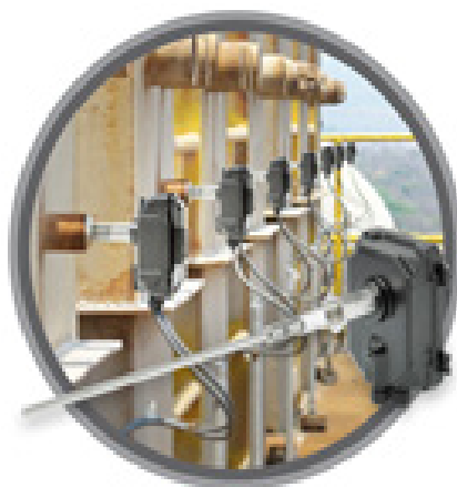
ENVEA ElectroDynamic™ sensor installation for multi-compartment baghouse performance monitoring
