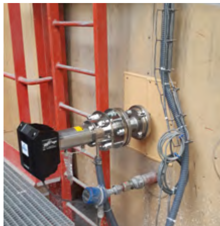
CROSS DUCT, INLINE COMBUSTION MONITORING
