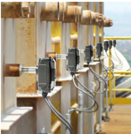
BROKEN BAG DETECTION WITH EXTERNAL DISPLAY
