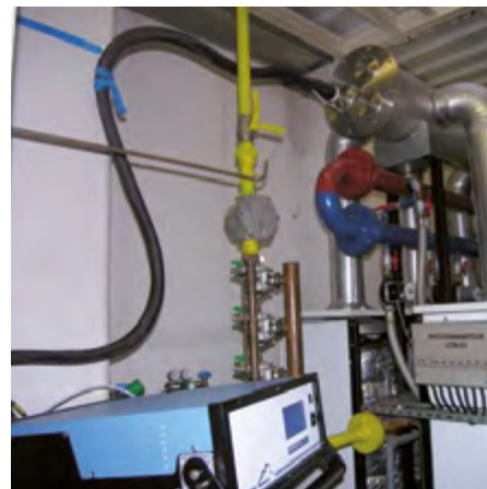
MONITORING OF COMBUSTION GASES ON INDUSTRIAL FURNACE
