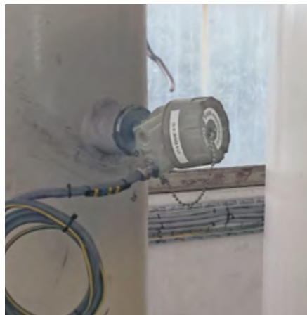
COMPACT SENSOR FOR BROKEN BAG DETECTION
