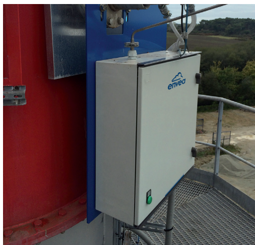
Sampling cabinet: Includes flow, temperature and pressure measurement and interface for starting leak tests
